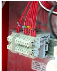
Alarm contact connections for Power Loss and Motor Run
