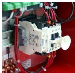
Alarm contact connections for Power Loss and Motor Run
